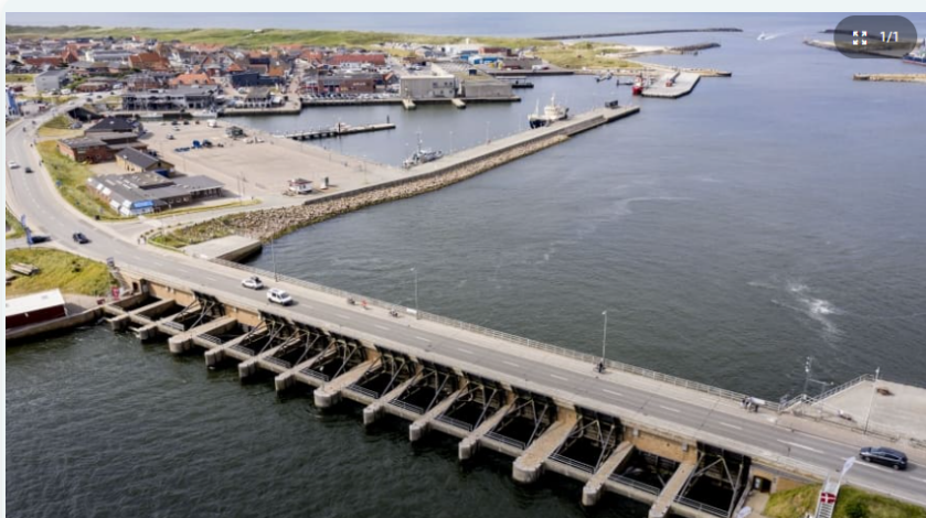
Pilot project approved for deployment in Hvide Sande Harbour
